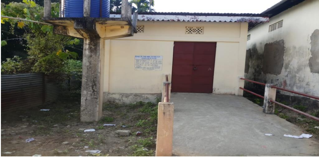
Divyangjan -friendly washrooms in the college campus
